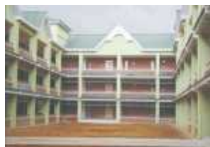
Temporary Academic Block at Shahpur
