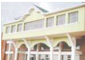
Temporary Academic Block at Shahpur
